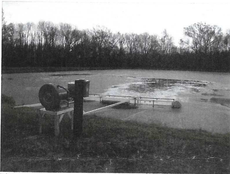
Figure 4: Diffused Aeration
