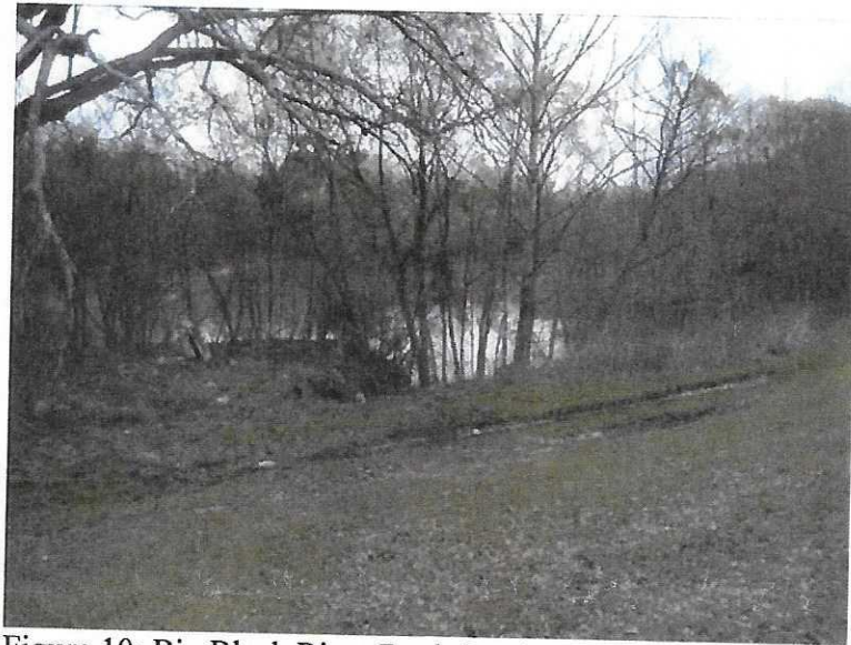
Figure 10: Big Black River Bank Erosion at the Facility
